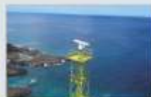
Coastal Surveillance System
